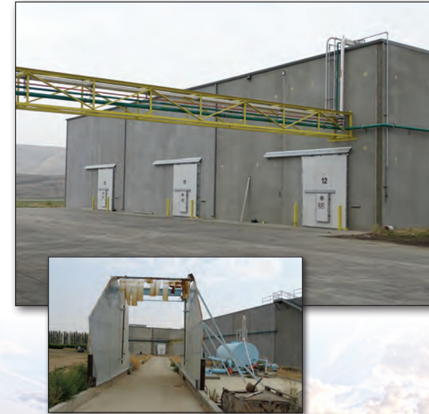
Controlled atmosphere storage buildings and drive-through drencher system.
